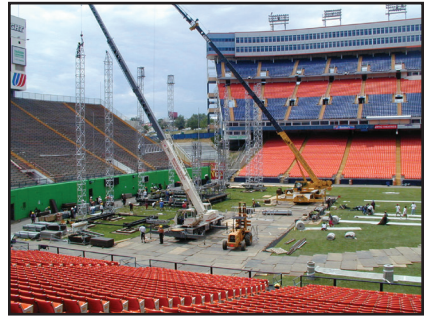
Set up for a concert showing field protective coverings. Photo: Ross Kurcab, CSFM
